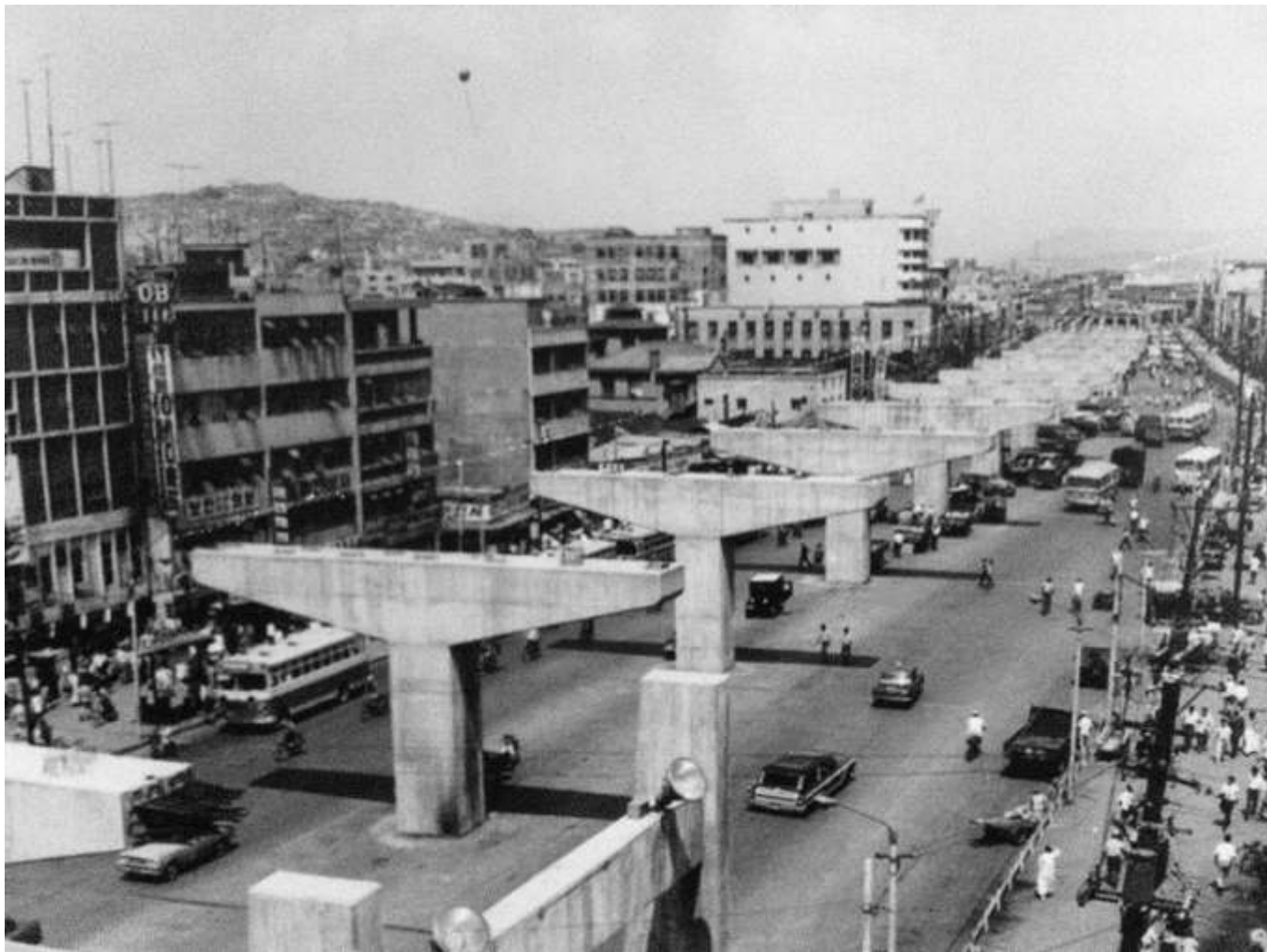
Seoul Cheonggyecheon motorway
